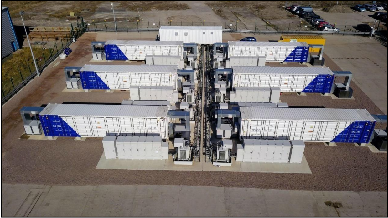
Photograph 1.2: Example of BESS located in storage containers
