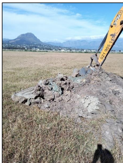
Figure 7-3: Residual shale excavation spoil material (left) and aeolian excavation spoil material (right)
