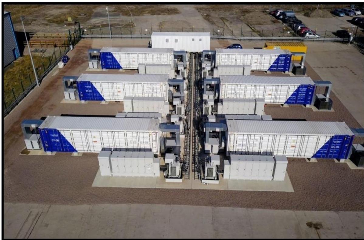
Figure 21: Example of a BESS in storage containers
