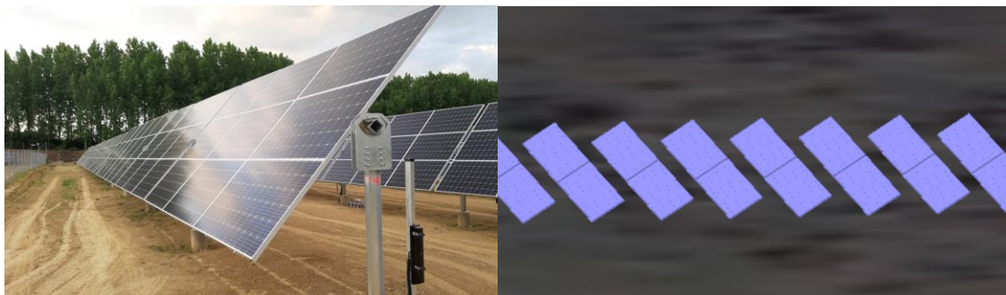
Figure 17: Paardevlei Solar PV Facility & BESS project - PV Layout 2 (Single Axis tracker panels)
