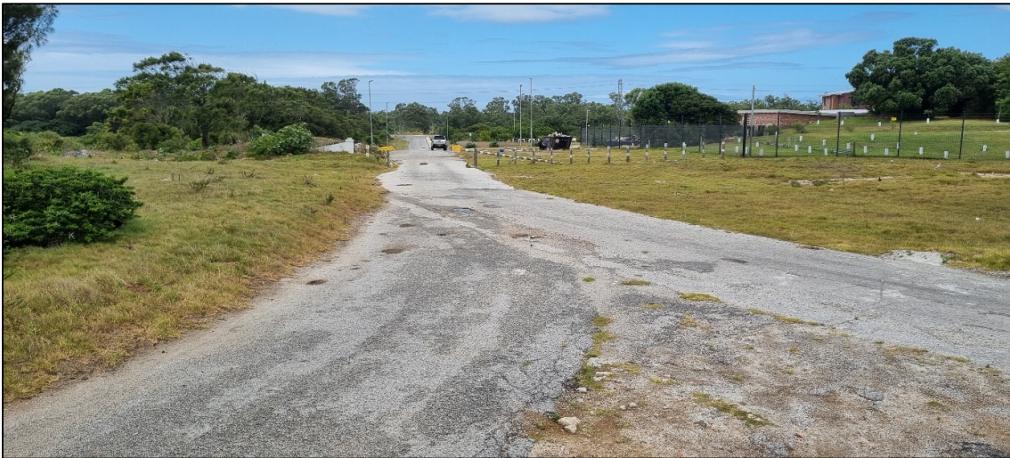
Figure 19. View of the entry / exit point to the property showing the location of proposed pipelines and pedestrian walkway.
