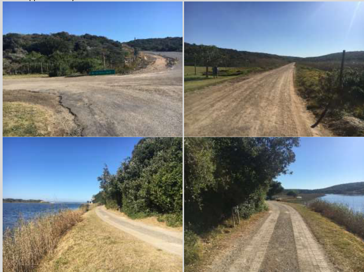
Plates 1 – 4: Photographs of existing access to the Riet River Access Road.
