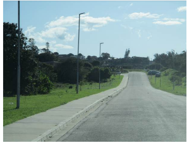
Surfaced sidewalk along the DR01908
