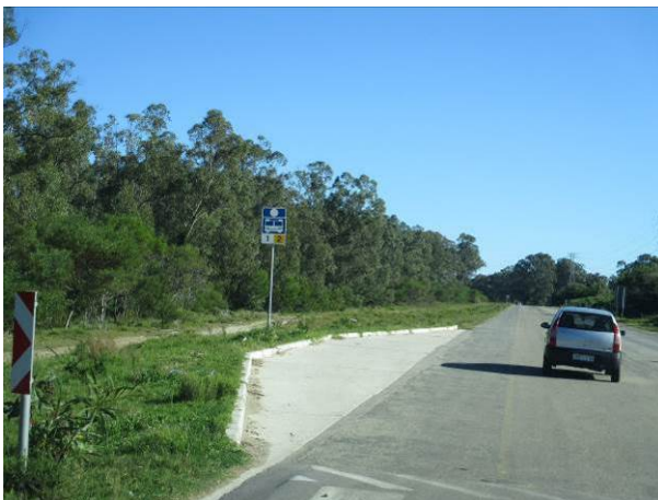
Victoria Drive/DR01908 (westbound) public transport facility
