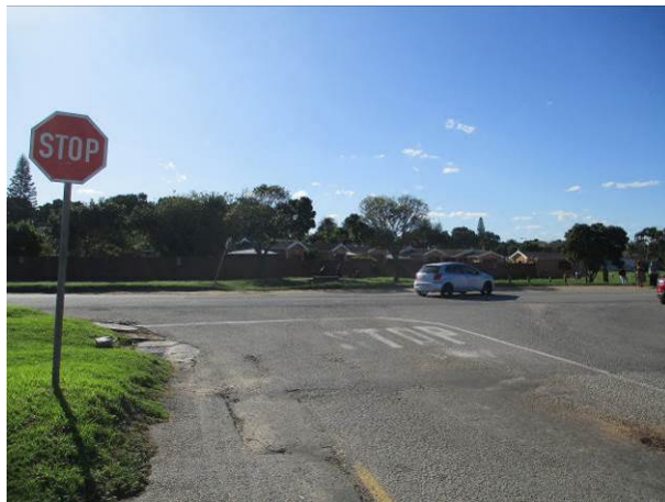
Genadendal Road/Buffelsfontein Road intersection
