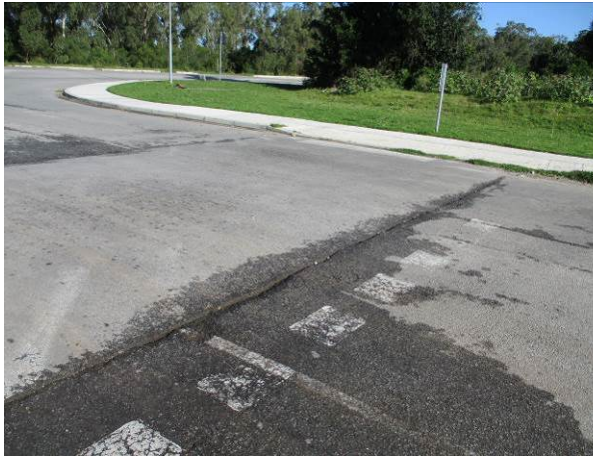
Raised pedestrian crossings at the Victoria Drive/DR01908 intersection
