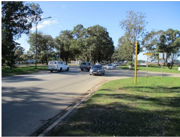
Buffelsfontein Road/Victoria Drive intersection
