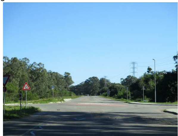
Traffic circle, with raised pedestrian tables, at the Victoria Drive/DR01908 intersection
